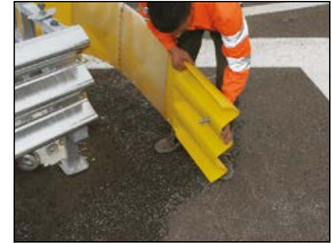
Figure 23 - Lock sliders
