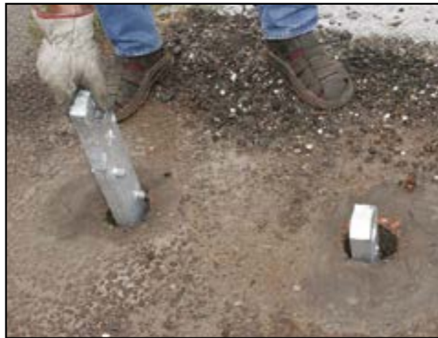
Figure 3 - Filling with chemical grout
