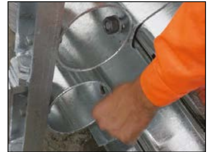
Figure 17 - Terminal beam positioning
