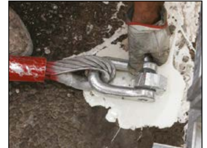
Figure 10 - Attach the cables to backup
