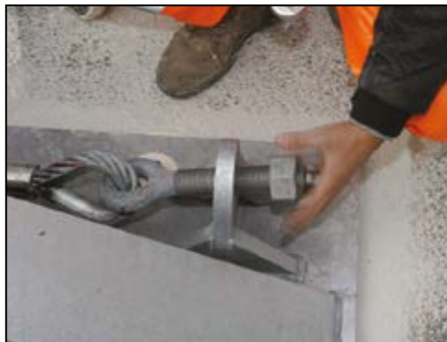
Figure 16 - Cable attached to the backup
