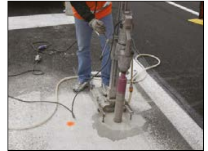
Figure 5 - Holes preparation for backup
