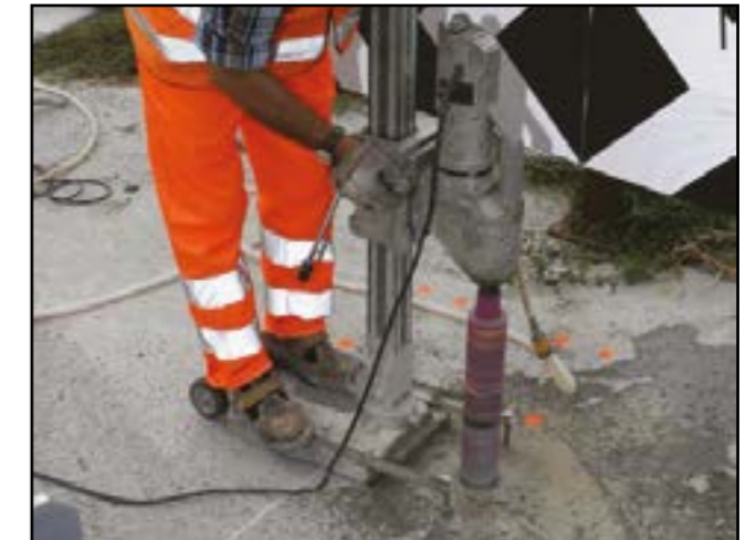
Figure 5 - Preparation holes for backup
