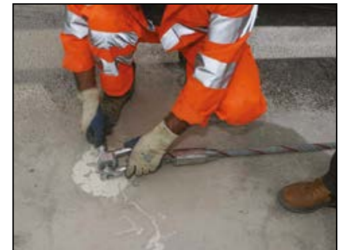
Figure 18 - Locking cables
