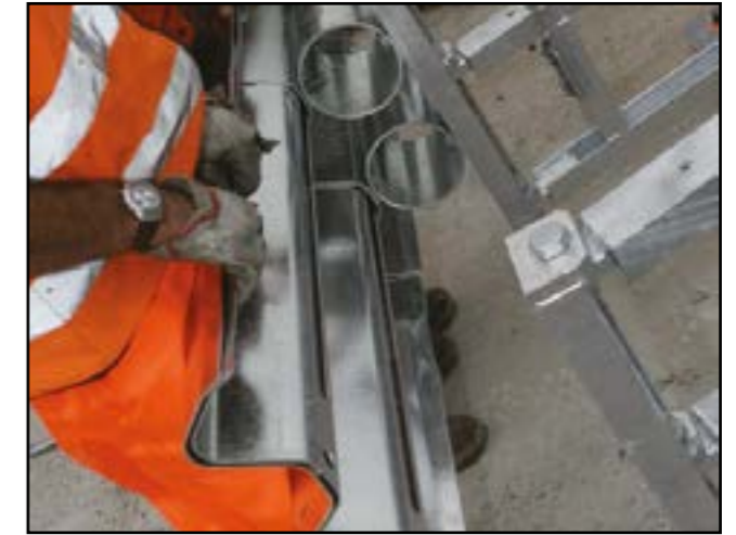
Figure 16 - Terminal beam positioning
