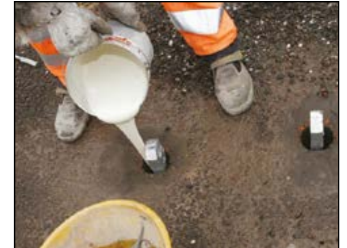
Figure 4 - Inserting pole anchor
