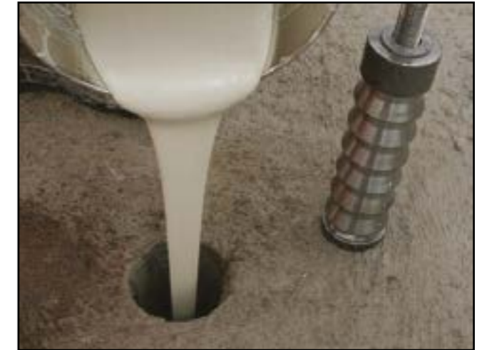
Figure 6 - Preparation holes for backup
