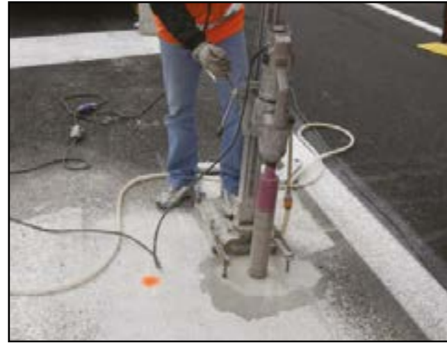
Figure 2 - Coring for the anchoring piles
