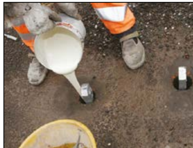
Figure 4 - Front picket insertion
