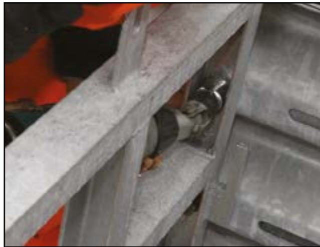
Figure 21 - Tightening of the sliders
