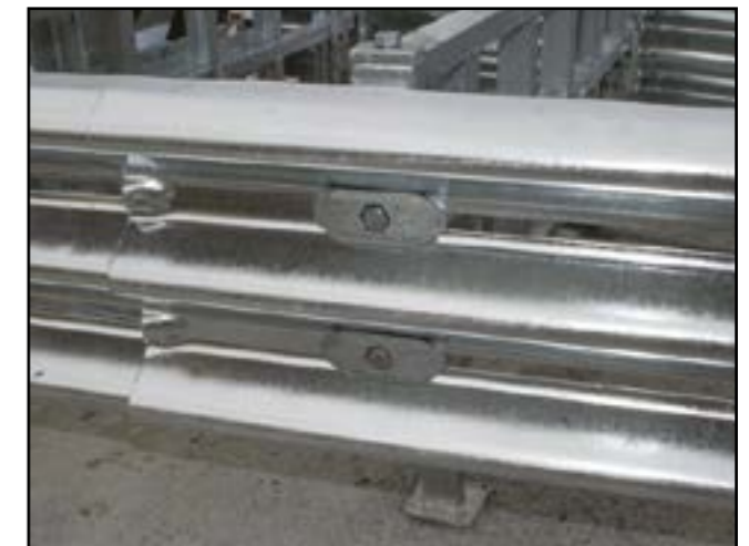
Figure 18 - Tightening screws sliders
