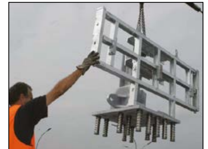
Figure 6 - Inserting fixing bars in the backup
