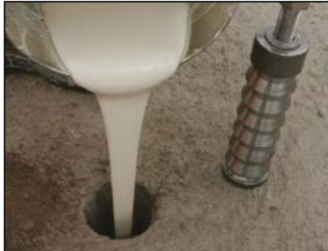
Figure 7 - Grout inclusion
