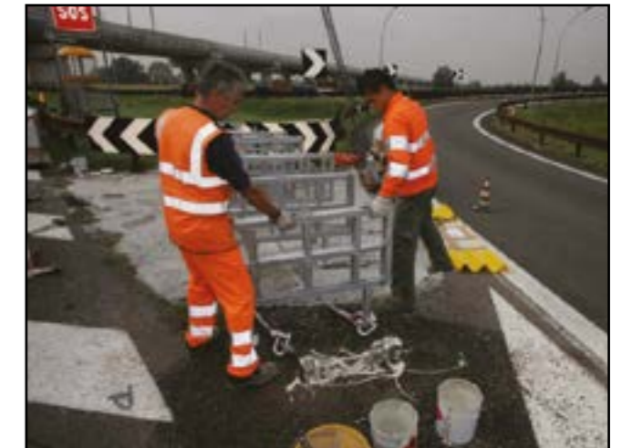
Figure 12 - Positioning of intermediate frames
