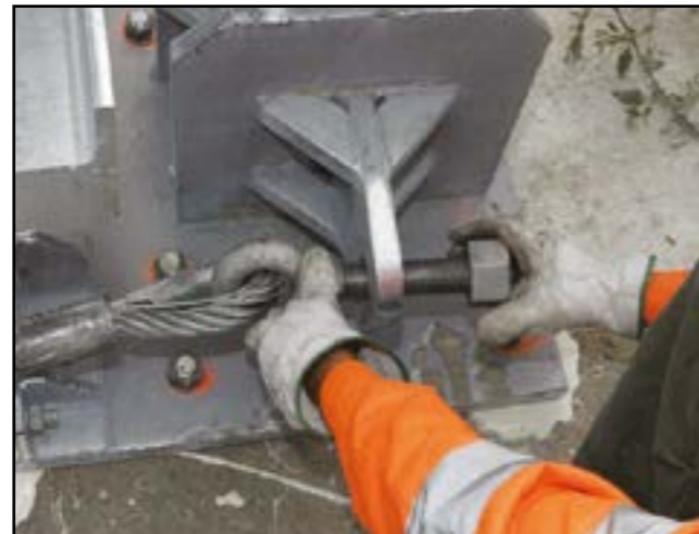
Figure 9 - Attach the cables to backup
