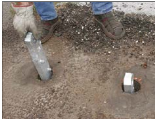
Figure 3 - Inserting pole anchor
