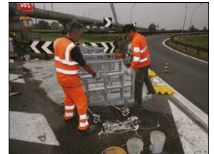
Figure 12 - Positioning of intermediate frames
