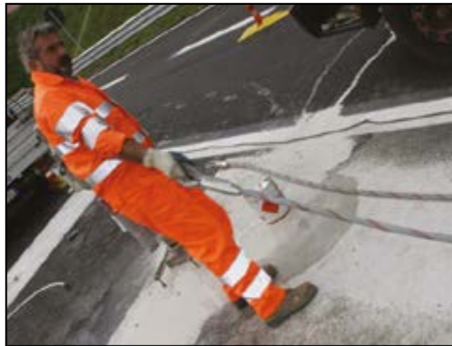
Figure 15 - Cable attached to the backup
