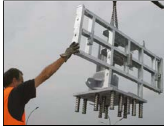
Figure 7 - Fixing bars insertion in backup
