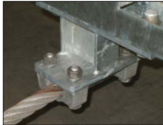
Figure 14 - Cables guide
