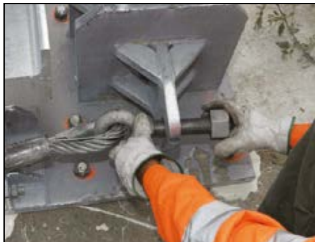
Figure 9 - Attach the cables to backup
