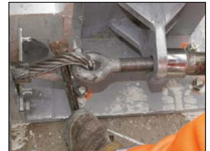
Figure 12 - Cable tensioning
