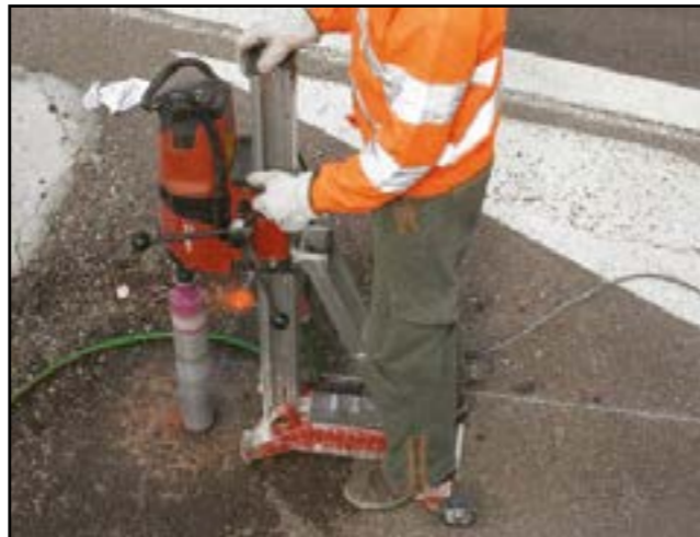
Figure 2 - Coring for the anchoring piles
