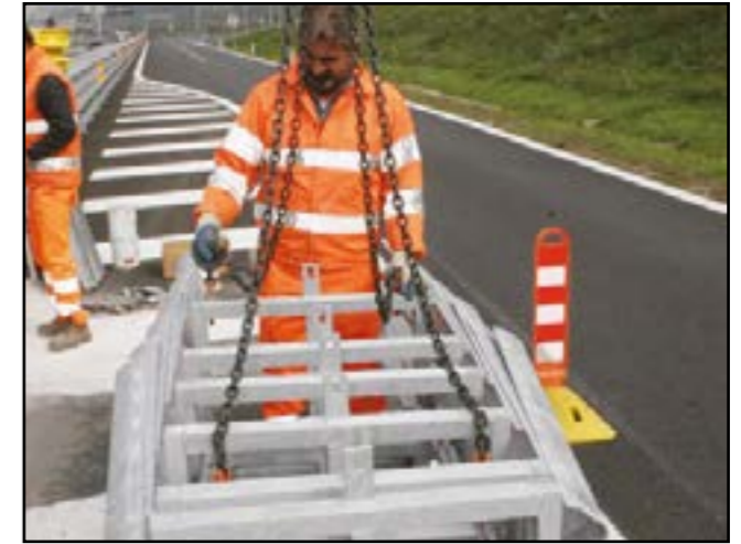
Figure 11 - The TAU® preassembled system positioning
