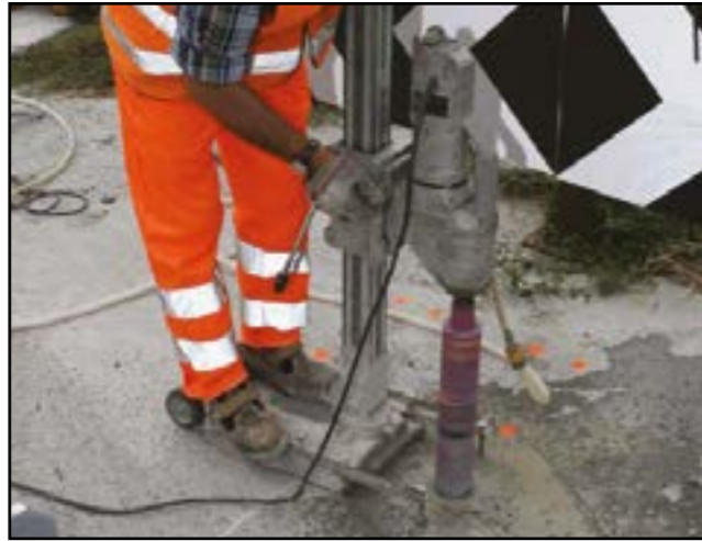
Figure 2 - Coring for front pickets
