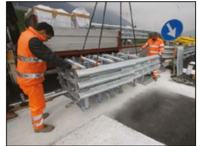
Figure 12 - The TAU® preassembled system positioning
