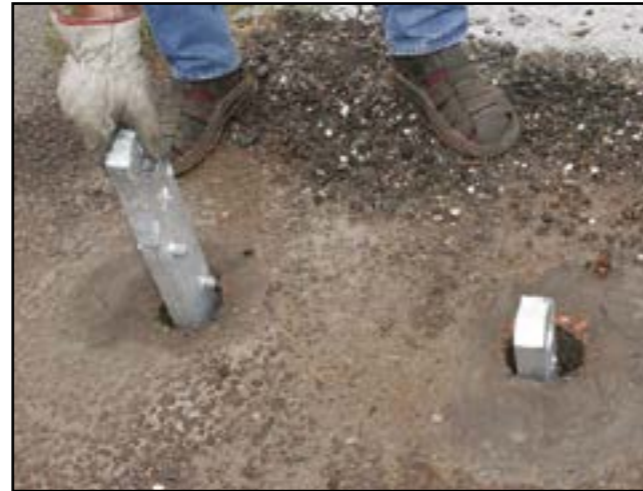
Figure 3 - Front picket insertion
