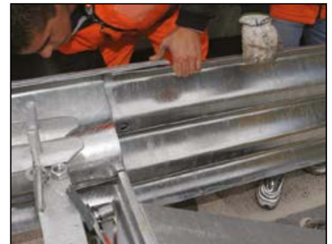
Figure 13 - Fixing of preassembled TAU®
