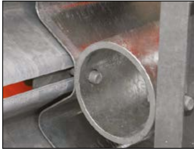
Figure 14 - Fixing of preassembled TAU®
