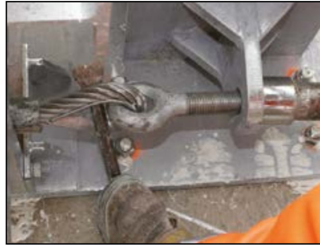
Figure 19 - Cable Tensioning
