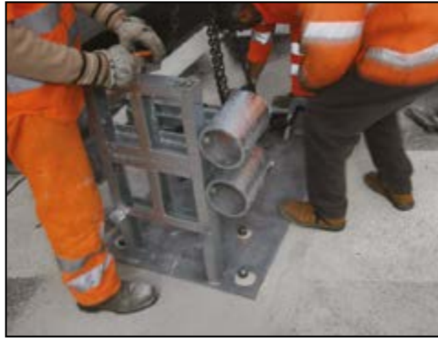
Figure 8 - Placement of the backup
