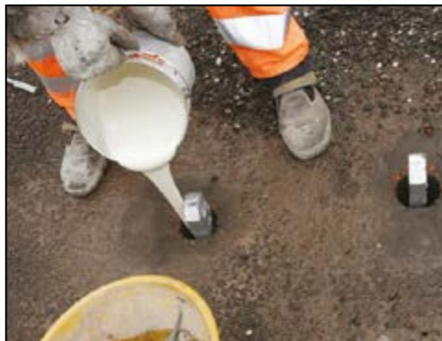
Figure 4 - Pickets inserting
