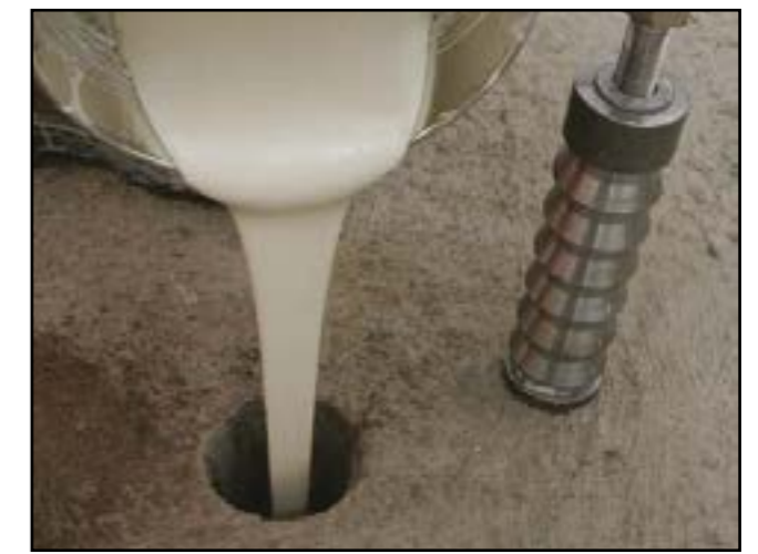
Figure 6 - Preparation holes for backup
