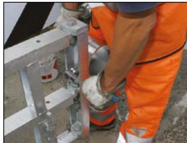
Figure 15 - Tighten the tube crosspiece
