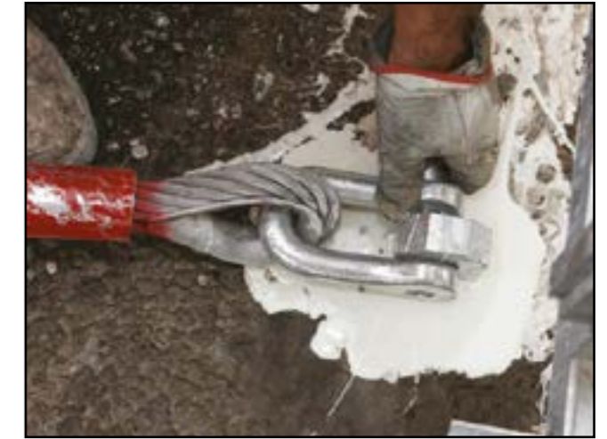
Figure 10 - Connecting cable to the front pickets
