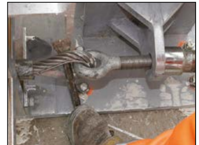
Figure 32 - Tensioning the cables
