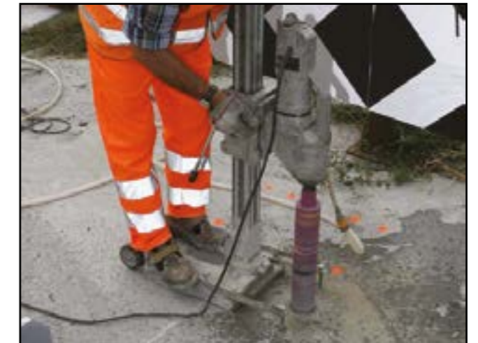
Figure 5 - Preparation holes for backup
