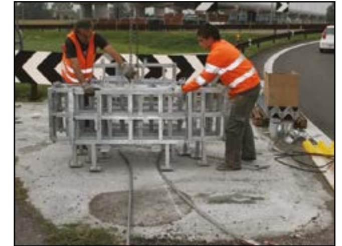
Figure 11 - Positioning of intermediate frames
