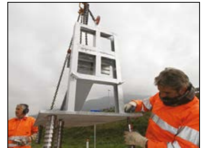
Figure 7 - Insertion of the fixing bars on the plate
