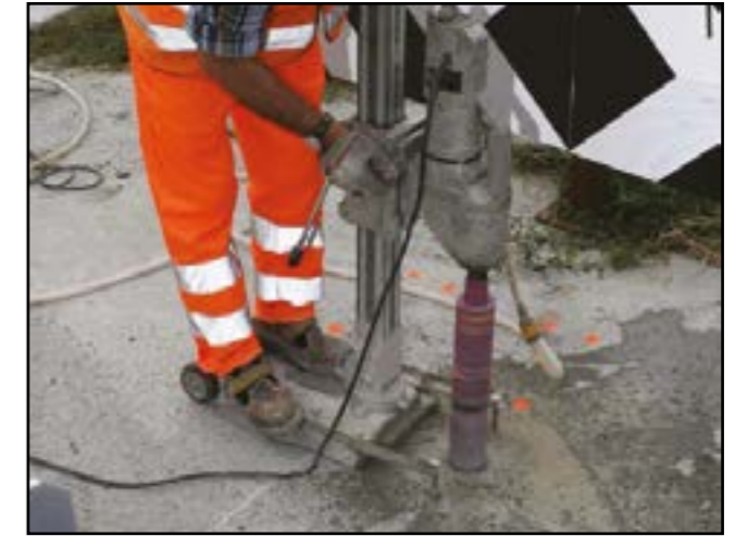
Figure 5 - Preparation holes for backup
