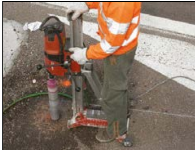
Figure 2 - Coring for the anchoring piles
